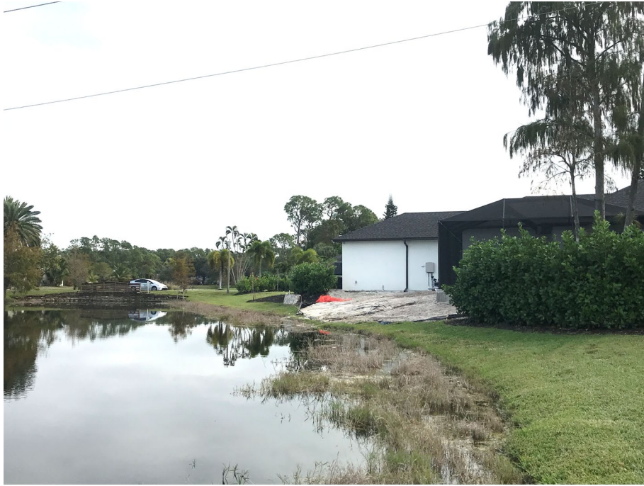
Photo 9: Lake 3 - View along the southern shoreline of Lake 3, note collapsed silt fence and fill material eroding down lake bank into lake.
